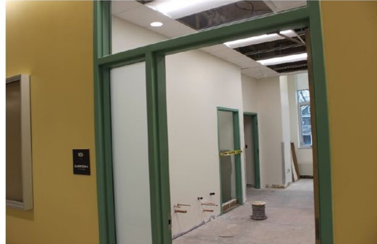
General interior progress- Rooms and gypsum board
