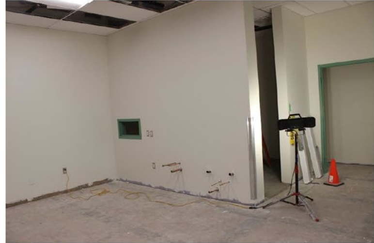
Mechanical awaiting fixture installation
