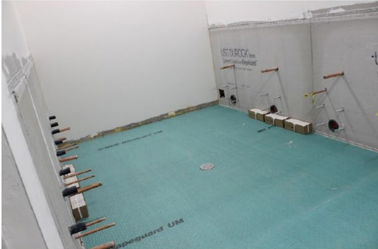
Preparation for tile flooring and mechanical fixtures
