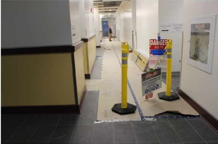
Interior Corridor- Signage and protection
