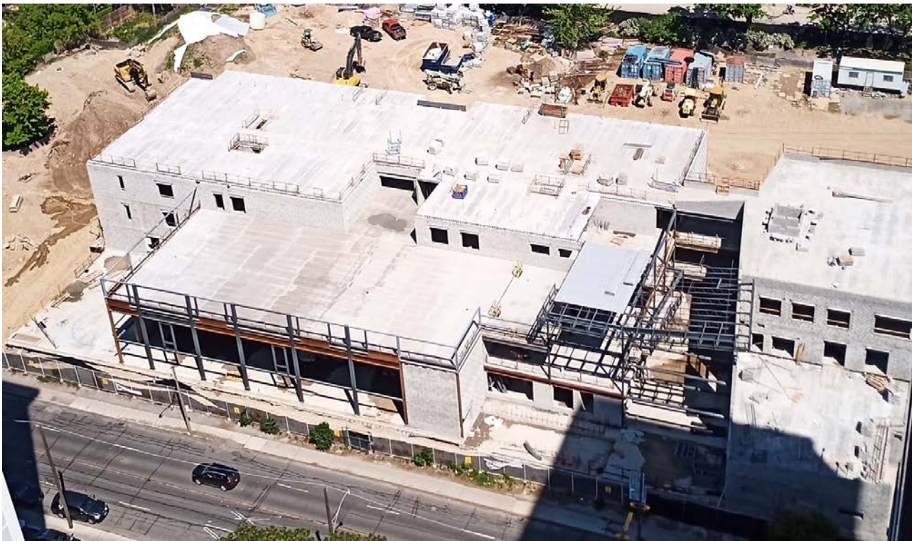
STATUS OF CONSTRUCTION – 7 June 2020
