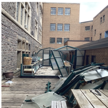
Greenhouse collapses under heavy snow
