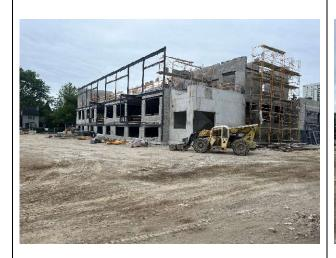
Exterior photo looking southwest at the new addition showing new exit stair to underside of 3<sup>rd</sup> floor and structural steel installation on the east elevation.
