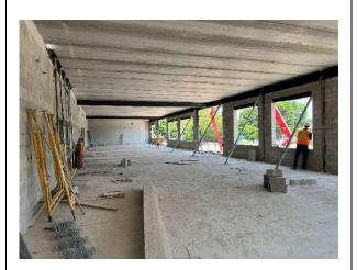
Interior photo looking to the north of the new 2<sup>nd</sup> floor classrooms showing load bearing masonry and structural steel progress.
