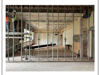
Interior photo looking east in existing library showing temporary shoring in place and masonry wall removed waiting for new steel beam installation.
