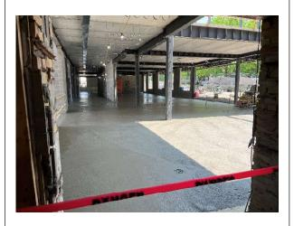
Interior photo looking to the east of new 1<sup>st</sup> floor corridor adjacent to new general office/main entrance showing placement of new slab on grade.
