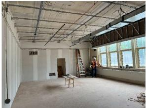
Interior photo looking northwest of existing tech room showing new subfloor installation, drywall, sprinkler piping and HVAC ducting progress.
