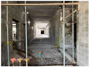
Interior photo looking to the west of new 1<sup>st</sup> floor corridor adjacent to new general office/staffroom showing completed underground rough-ins, stone subgrade placement and awaiting installation vapour barrier prior to slab on grade pour.
