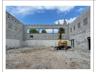
Interior photo looking to the north end of the new gym showing awaiting roof joist installation.
