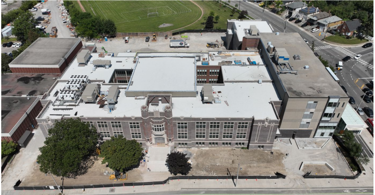
Zones A and B – Photo looking north through reinstated building.
