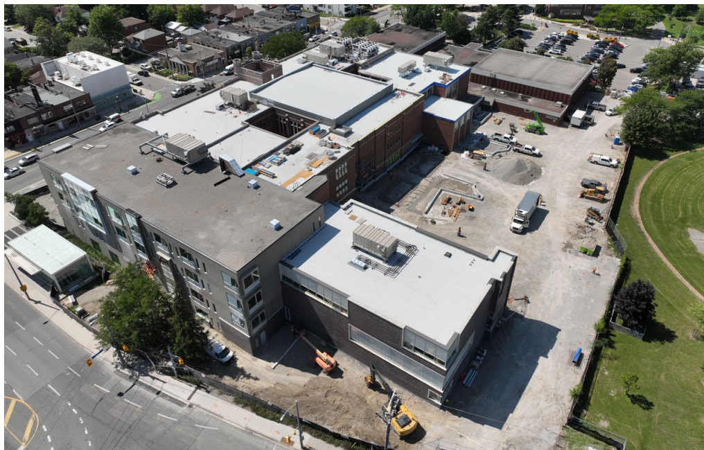
Zones A, B, and C – Photo looking south-west through reinstated building.
