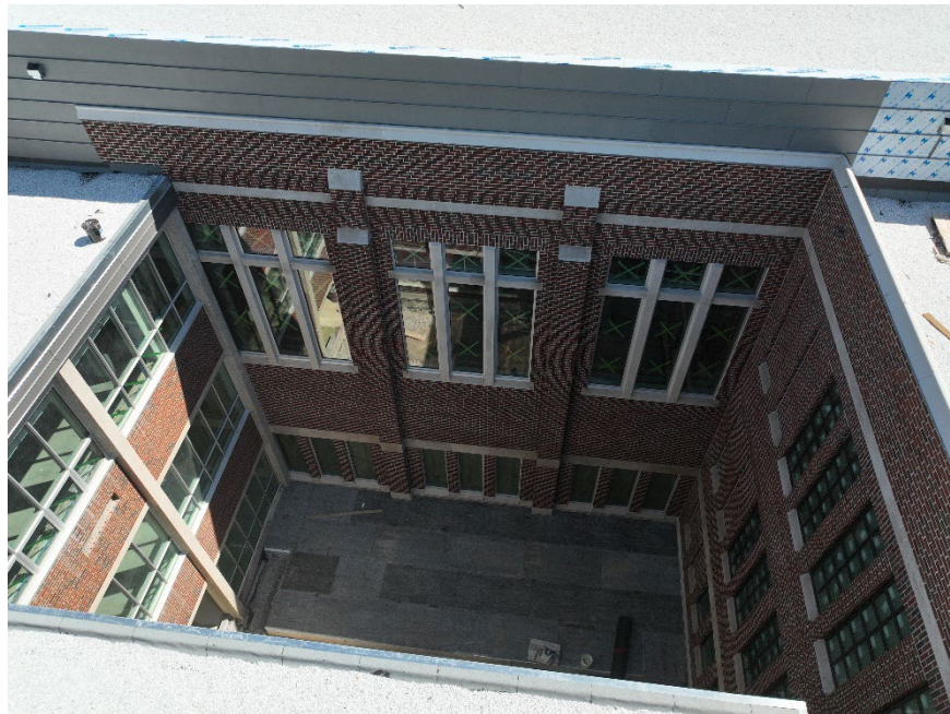
Zone A – Reconstructed Courtyard with new windows.
