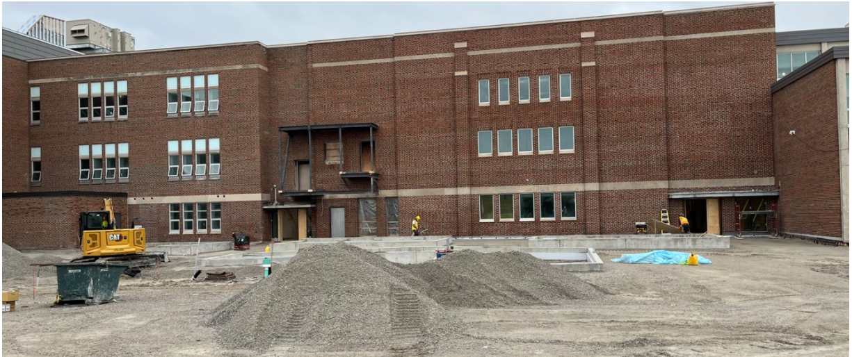
Zone A – Photo looking south through finished façade construction and ongoing landscaping.
