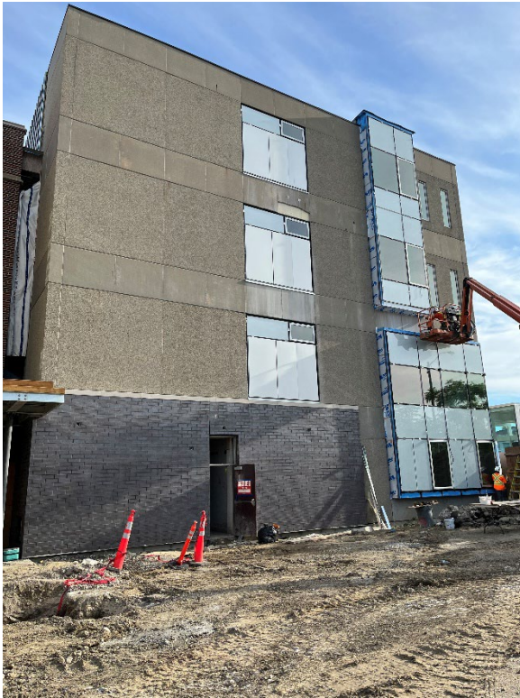
Zone B – Photo looking south and west at new façade and window installation.
