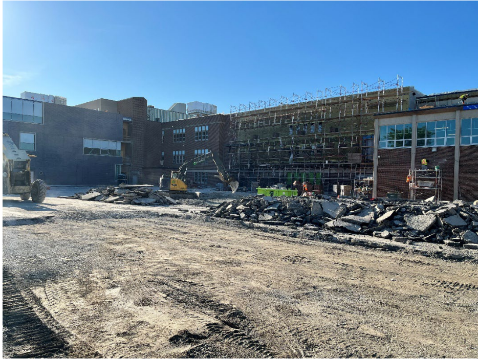
Zone A and C – Photo looking south-west through ongoing landscaping and façade reconstruction.
