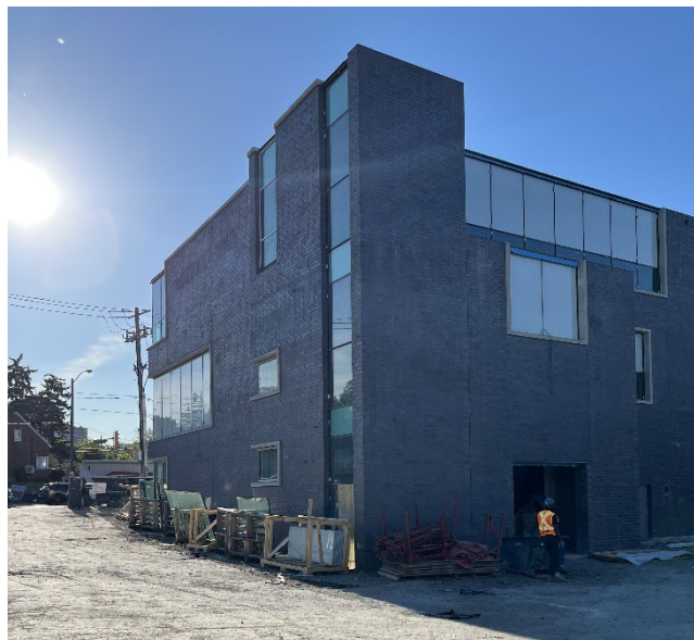
Zone C – Photo looking east at new façade construction.
