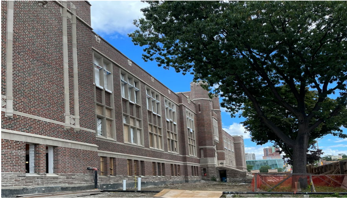
Completed south façade period masonry rebuild – ZONE A
