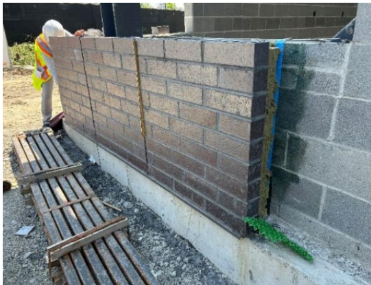
Masonry veneer mockup – ZONE C
