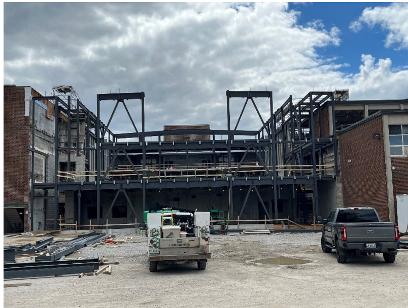
An overview of the auditorium steel installation – ZONE A
