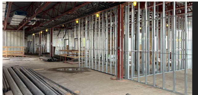
New steel stud installation – ZONE B
