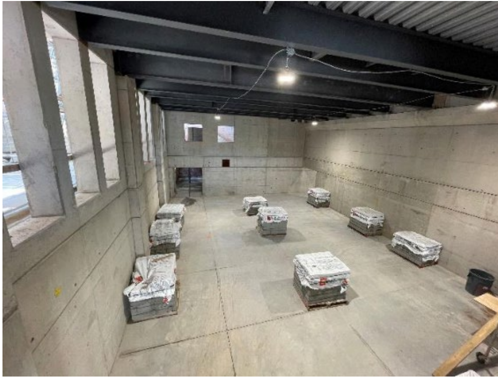
East new multipurpose room complete concrete slab – ZONE A
