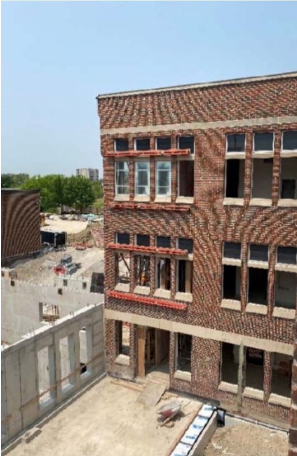
Window removals in progress to accommodate new operable windows. – ZONE A
