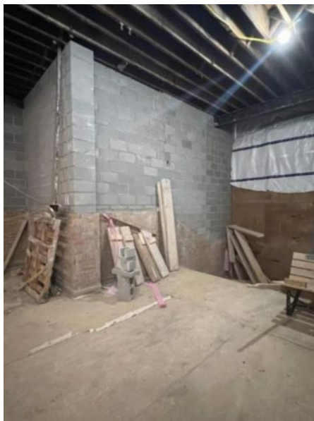
Completed second floor interior foyer brick and block work – ZONE A
