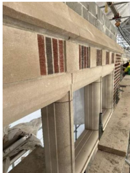
Third floor south exterior façade heritage masonry reinstatement – ZONE A
