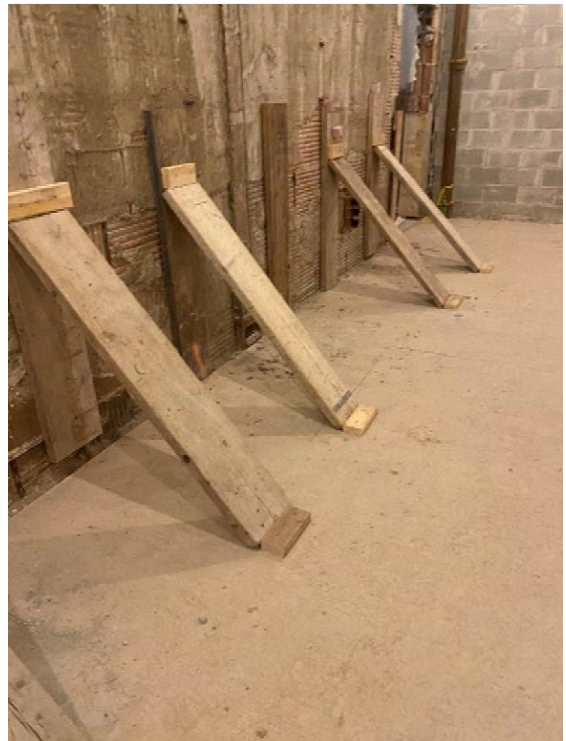
Heritage buff brick retention system – ZONE A
