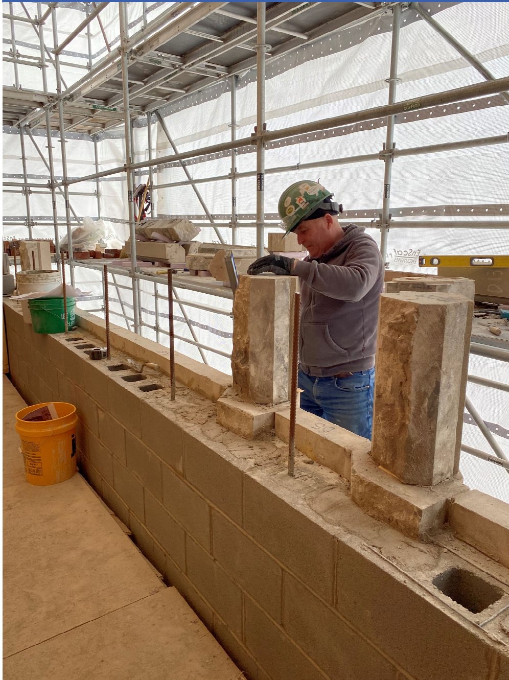
Restoration of the 1929 front façade east bay.
