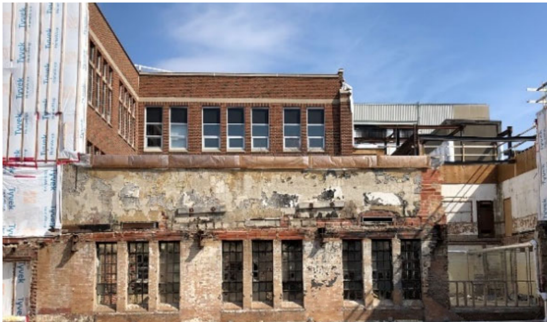
Post-fire view of dismantled east auditorium wall.
