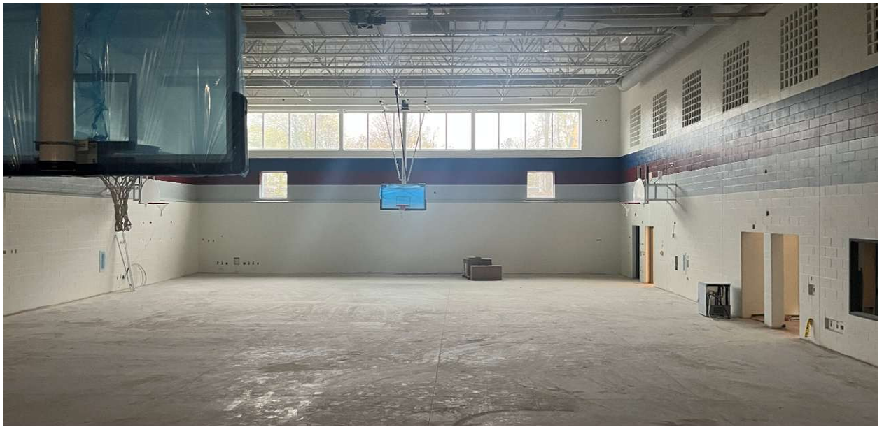
New Gymnasium progress.
