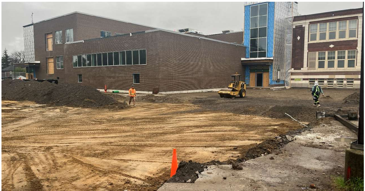
Exterior envelope & parking lot progress.
