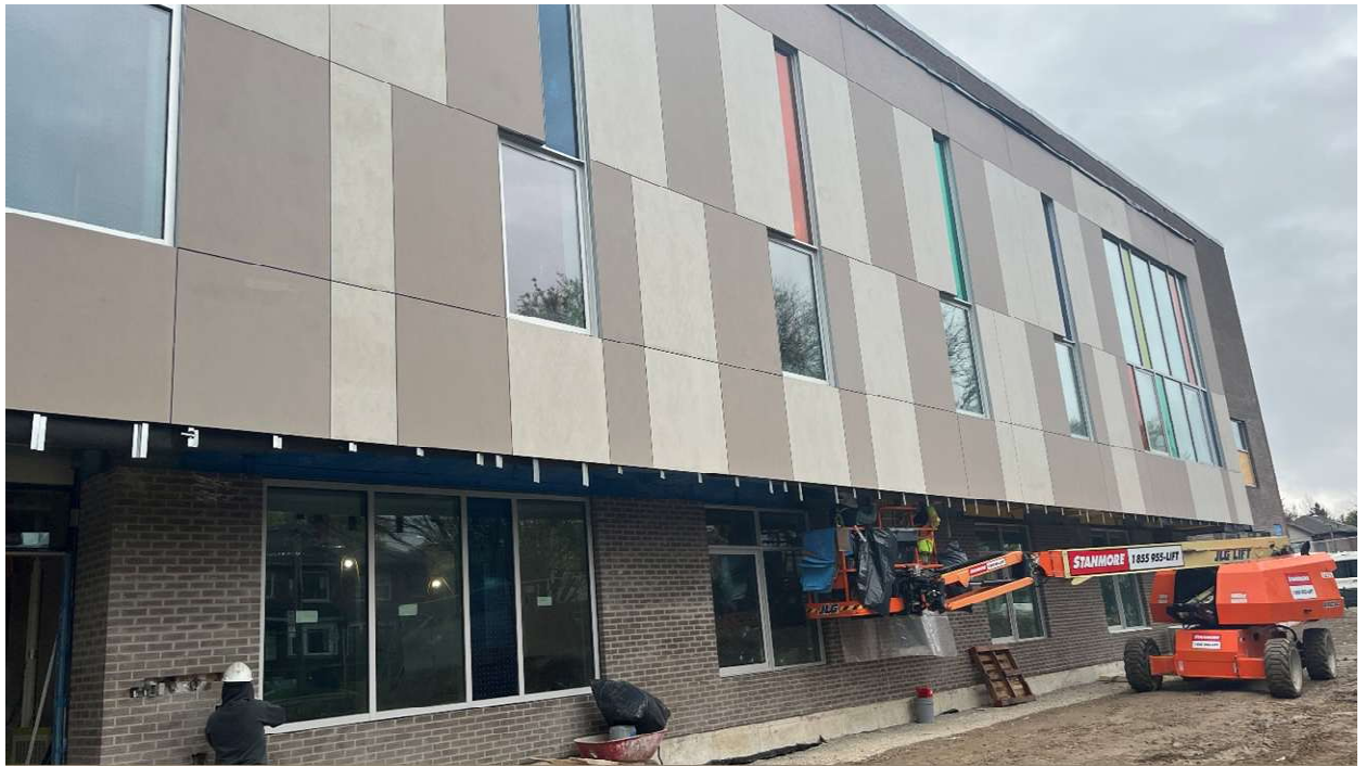
Exterior building envelope progress on south elevation of the new addition.
