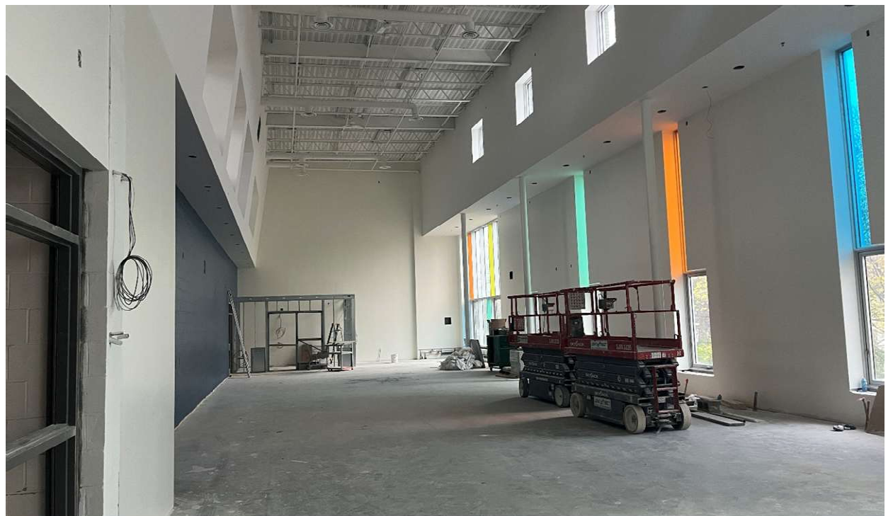
New Library progress.
