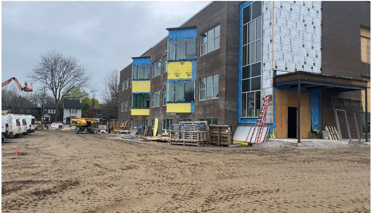
Exterior envelope progress.
