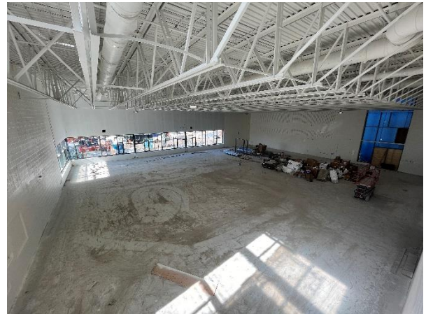
Picture from the Computer Engineering room looking down into the gymnasium. Ceiling and walls were recently primed.
