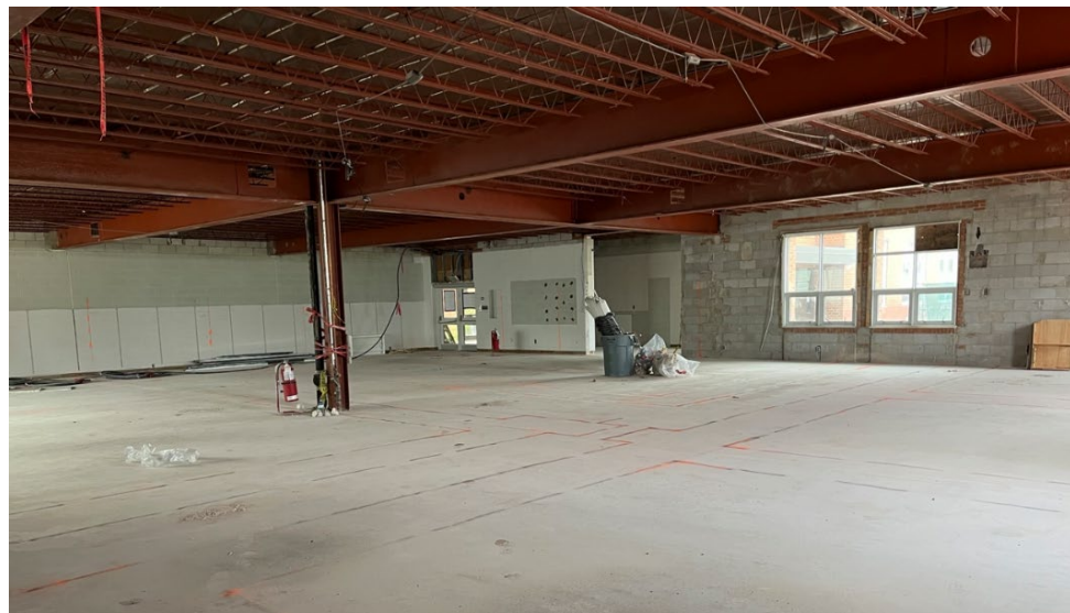
New Addition – Photo looking south-west through demolished interior of former library.
