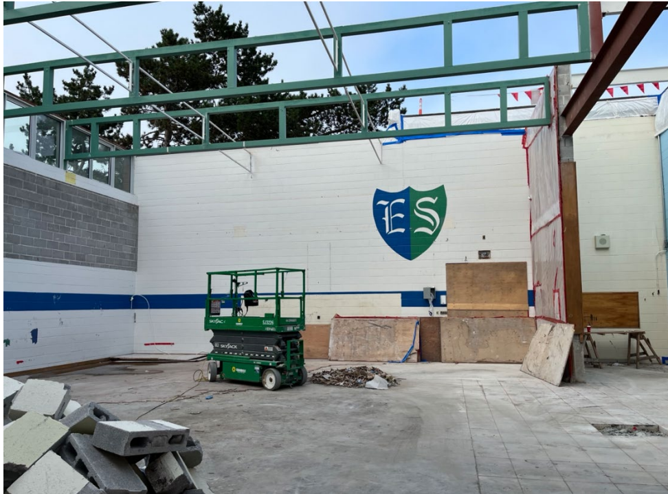
West Gym – Photo looking west through west gym of removed roof and stage.
