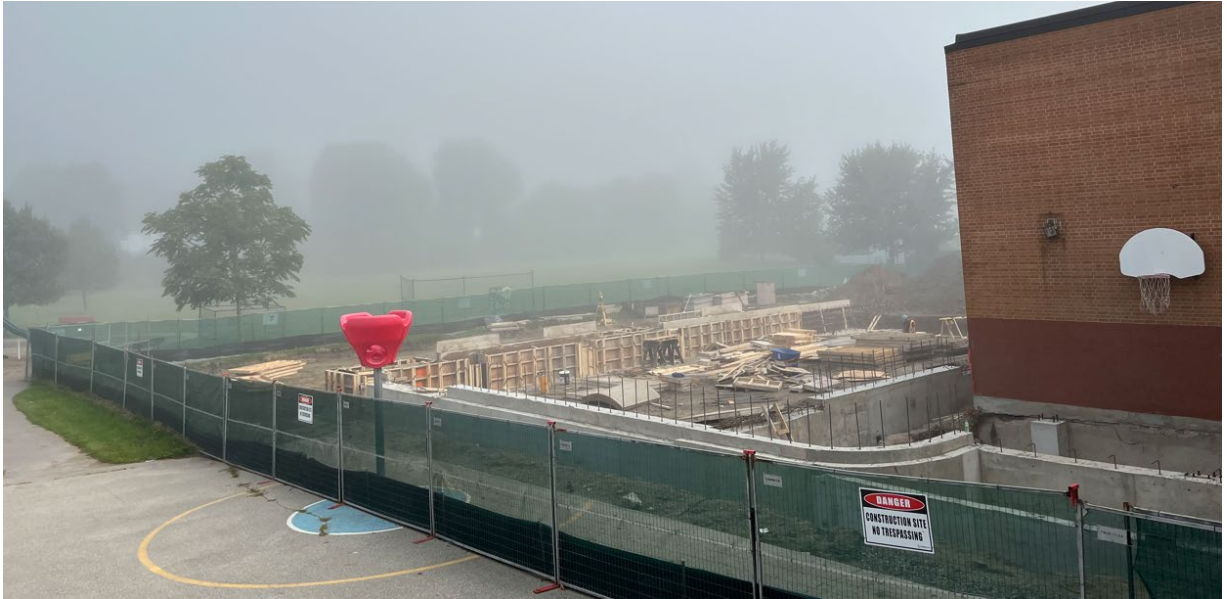
New Addition – Photo looking north through forming of foundations and footings
