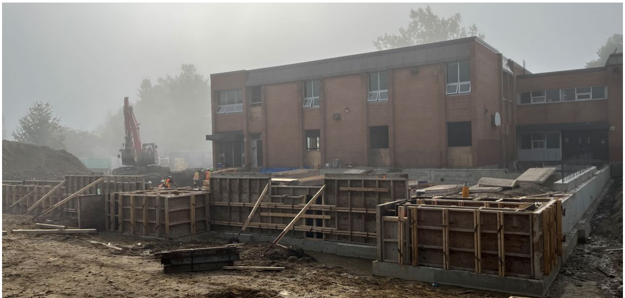
New Addition – Photo looking south at ongoing demolition and form work.
