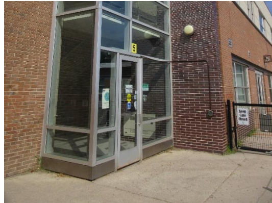
Staining/rust at grade- Aluminum doors & steel columns
