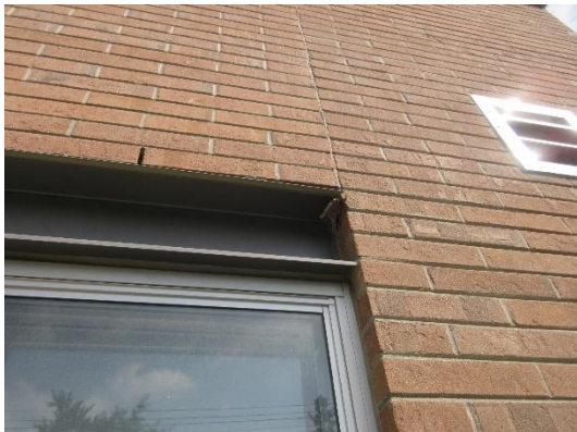
Exposed steel columns & Beams as window surrounds
