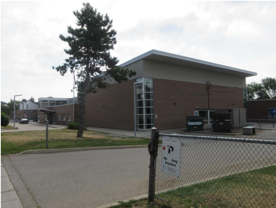
North- West Facade- Gymnasium & Parking Access
