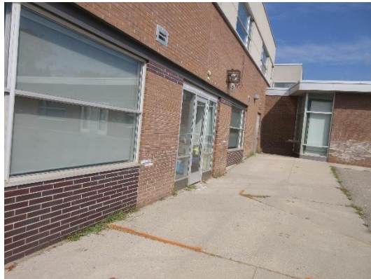
Staining/rust at grade- Aluminum doors & steel columns
