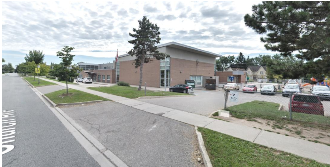
McKee Public School- Existing Building
