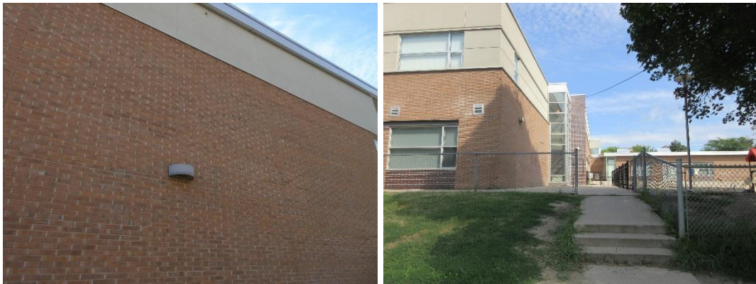
Stucco finishes at second floor in good condition
