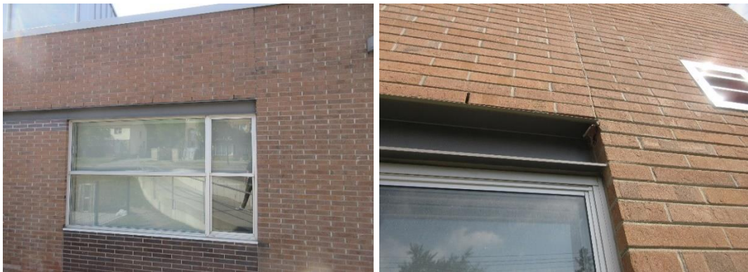
Aluminum windows in good condition
