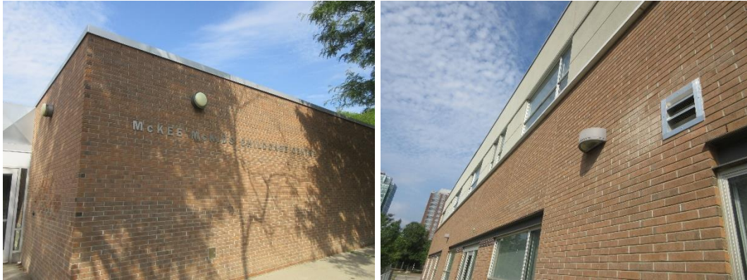
2 different types of wall sconce fixtures found at the site
