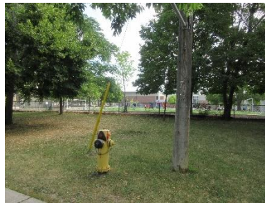
Dorris Ave. hydrant
