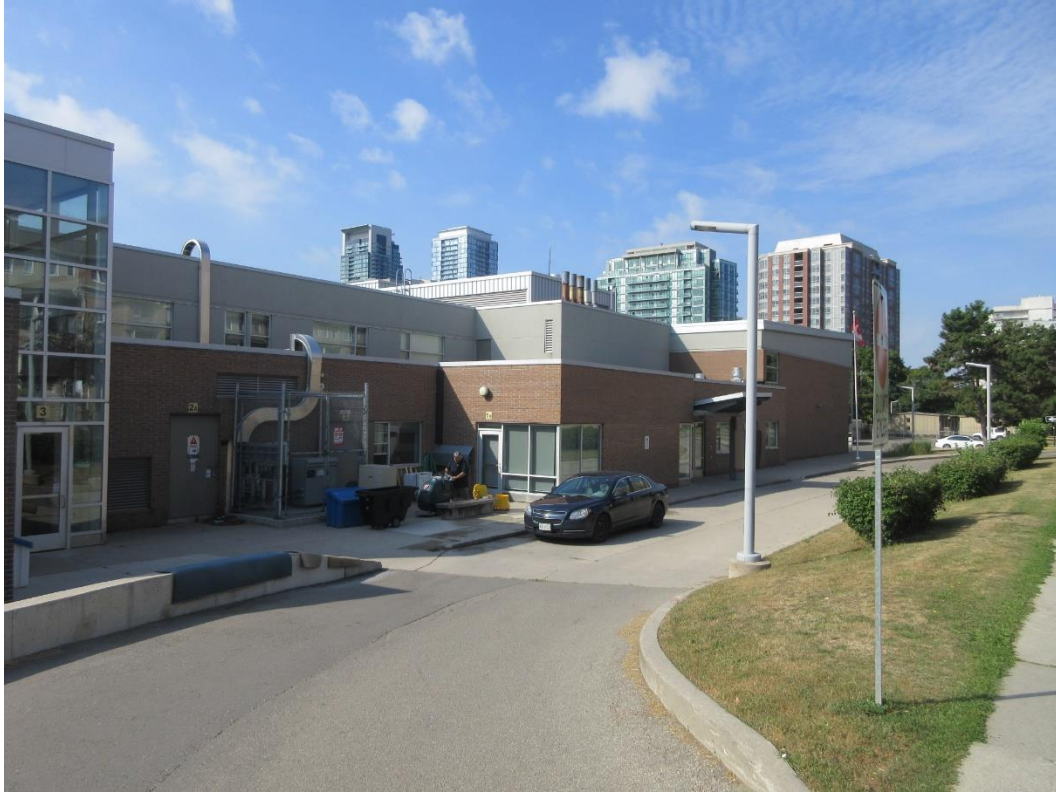
North Façade –Receiving doors & Fire route
