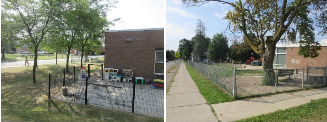
Chain-link fencing utilized throughout site
