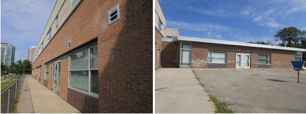
South façade- Child Care & Regular Classrooms
