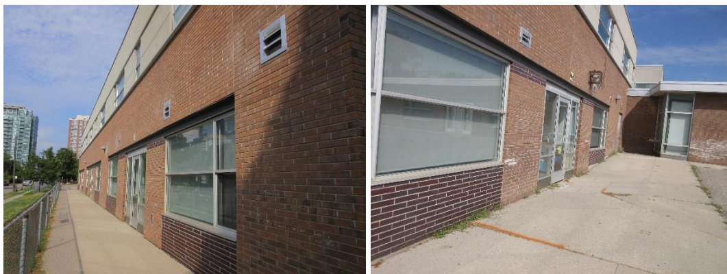
Exterior doors exit at grade onto flat level pathways
