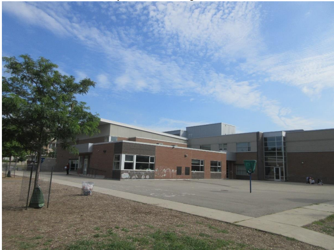
South-West corner- 2015 Addition area
